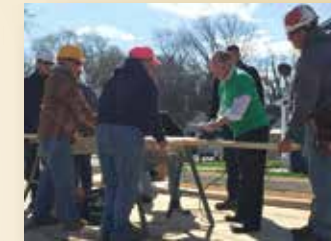
Building with Habitat for Humanity
